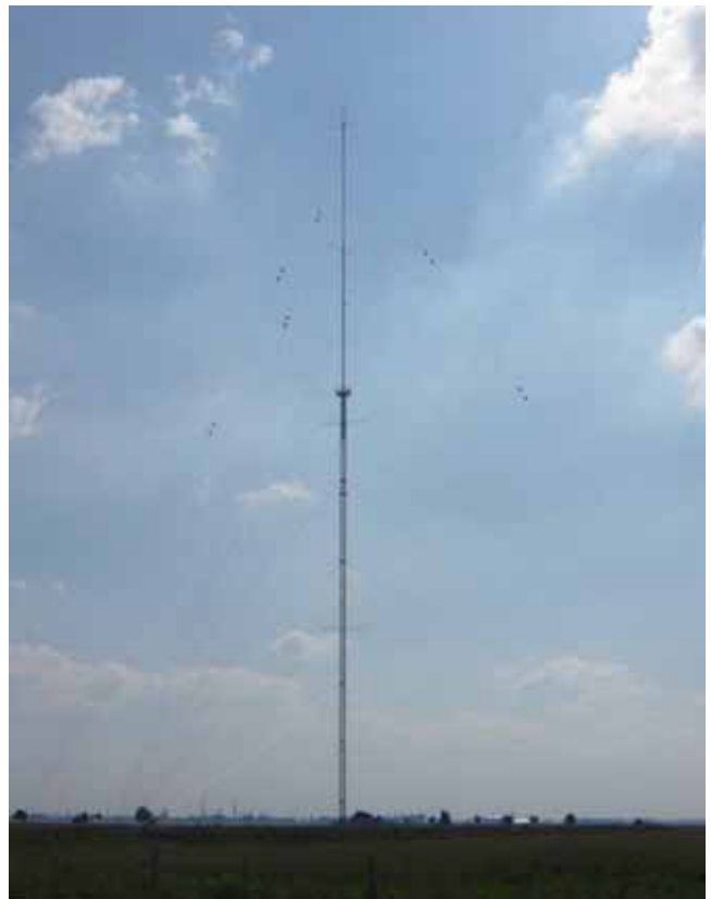
Photo 5: Measurement Tower 120 m
